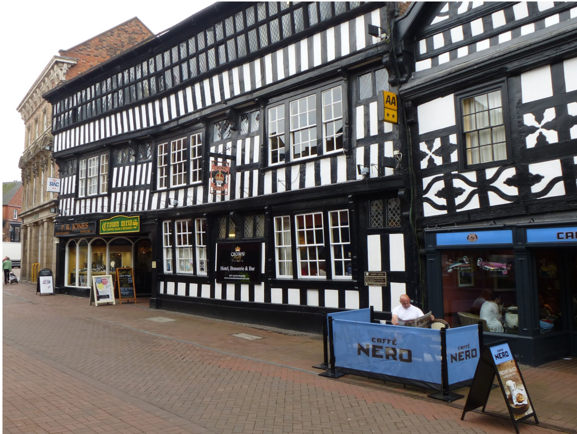
Crown Inn, High Street, Nantwich, Cheshire.
