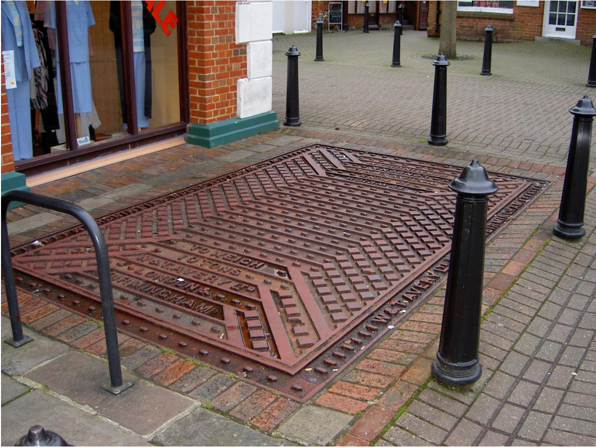
Illus. 3. Weighbridge. Market Square, Alton, Hampshire.
